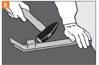
The last row of planks is rounded on the side with the pull bar and on the front side with the ZIRO tapping block.
